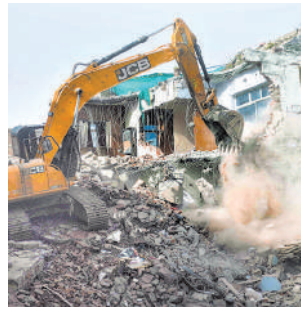
A house being demolished in Prayagraj. ■ PTI
